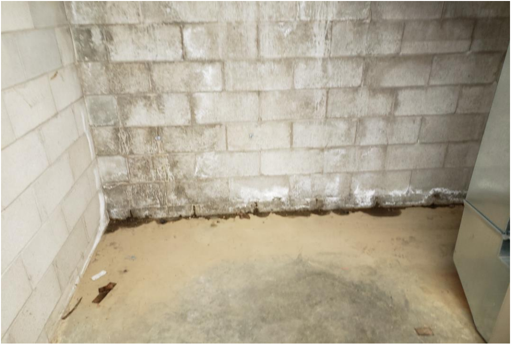
Photo 8: Location: Basement – Exterior Wall Item: Water intrusion through concrete block wall.
