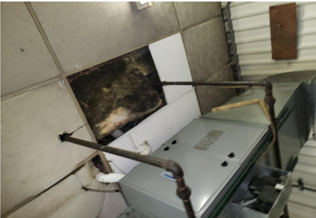
Photo 2: Location: Shop Area – Ceiling Item: Exhaust leak in furnace darkening the insulation.
