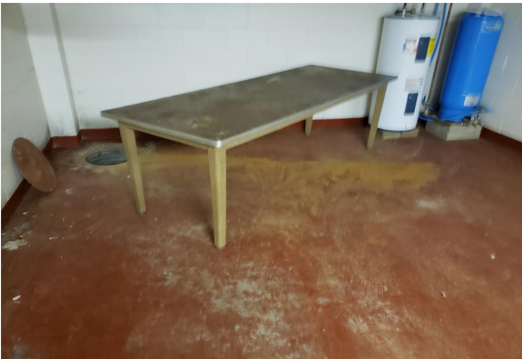
Photo 12: Location: Basement Item: Water staining on concrete floor from water intrusions.
