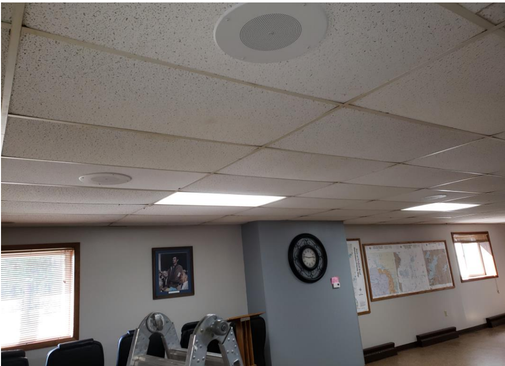
Photo 4: Main Level – Meeting Room Area Item: Overall View – Ceiling tiles sagging possibly due to previous humidity issues.
