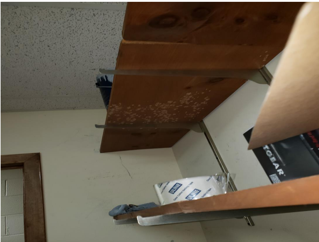
Photo 6: Location: Main Level – Office Item: Visible microbial growth on wood shelving unit likely caused by condensation.
