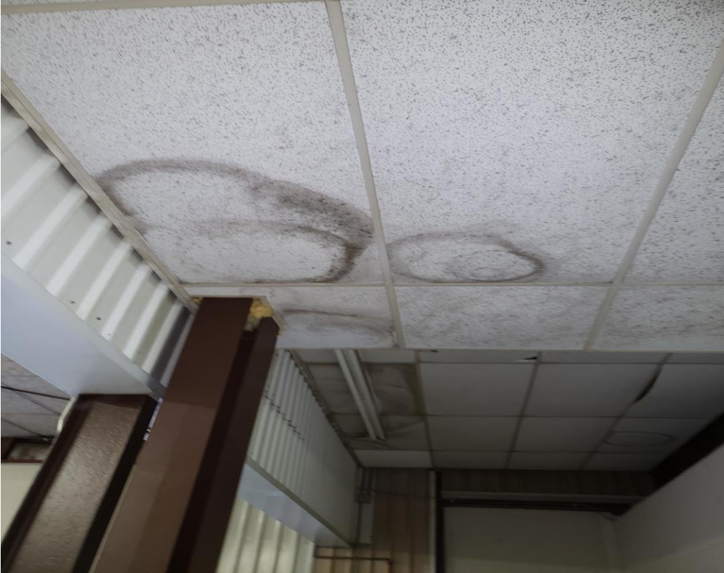
Photo 1: Location: Shop Area – Ceiling Item: Water damage on ceiling tiles from roof leak.
