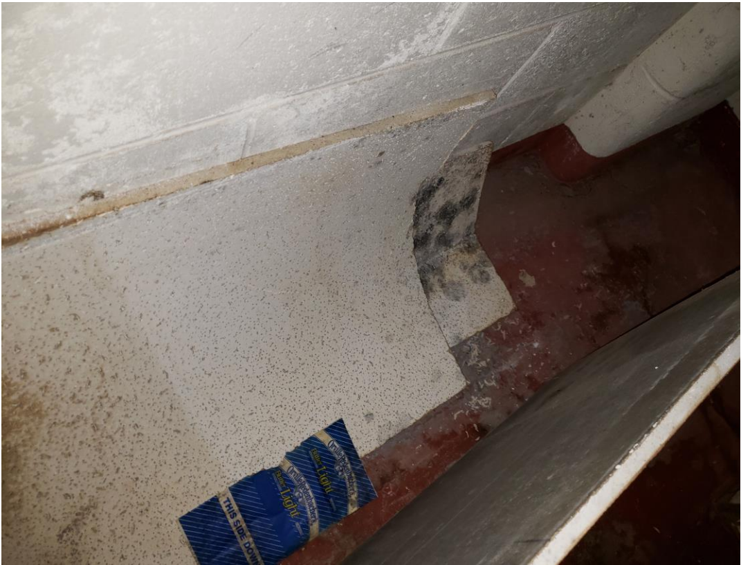
Photo 9: Location: Basement Item: Visible microbial growth on extra ceiling tiles.
