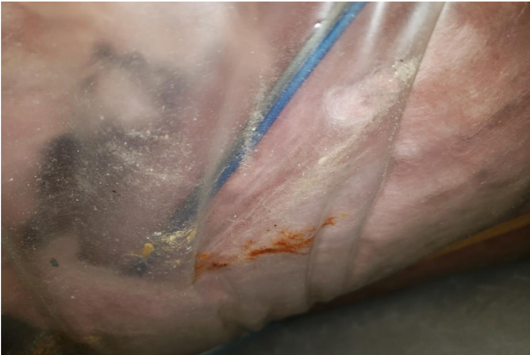
Photo 5: Main Level – Meeting Room Area Item: Water damage on insulation above ceiling tile.
