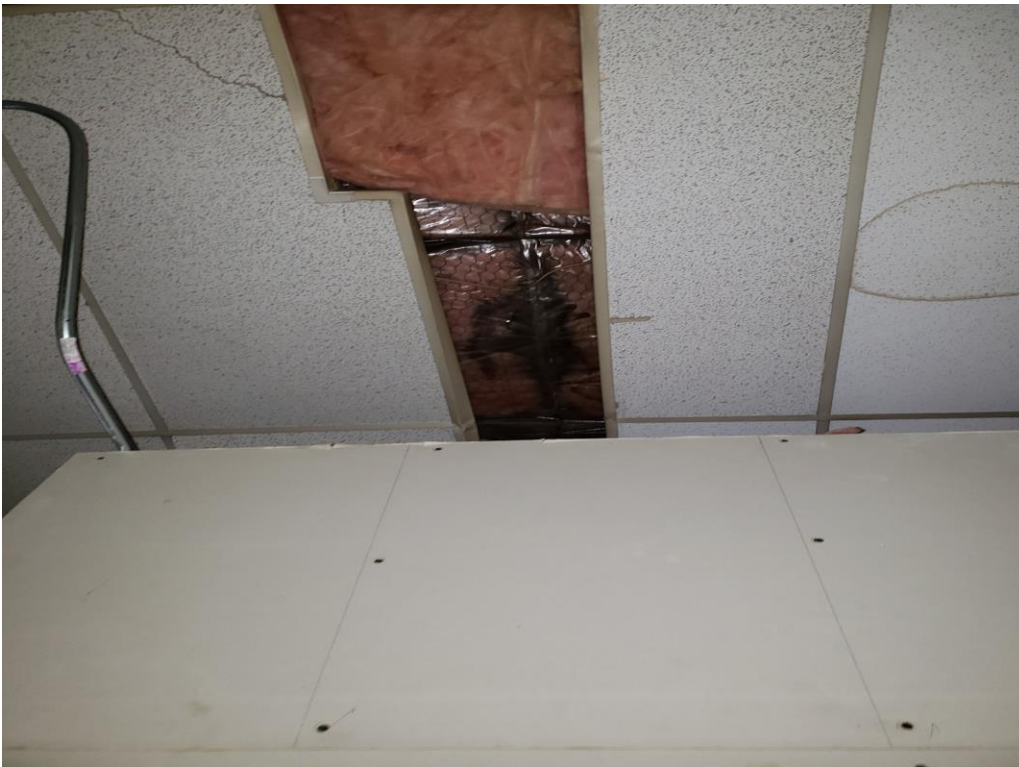
Photo 3: Location: Shop Area – Ceiling Item: Water damage on insulation above ceiling tile.
